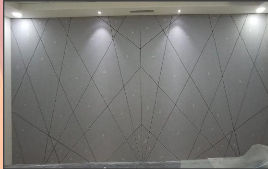
Walline Acoustics panel - CNC cutting
