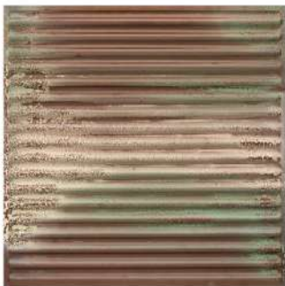
261 - Corroded Metal (V1)
