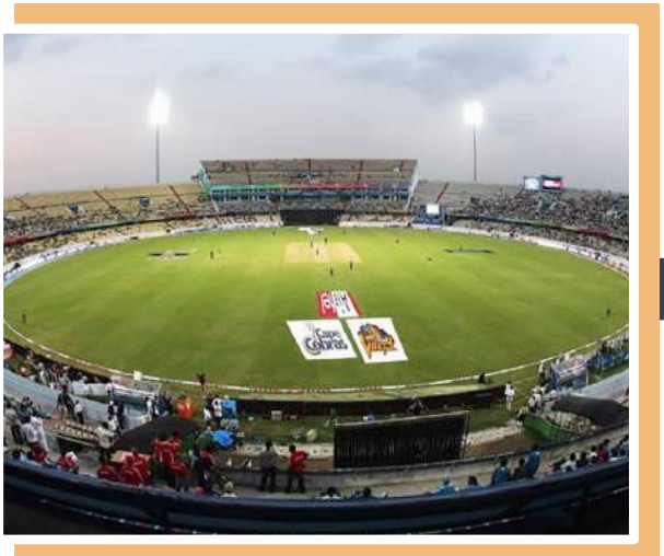
HYDERABAD STADIUM COMPLETE ROOFING WORK
