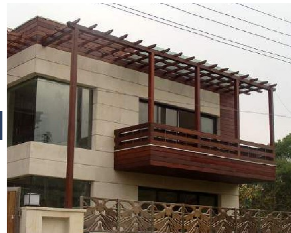
PRIVATE HOUSE PARGOLA, CLADDING
