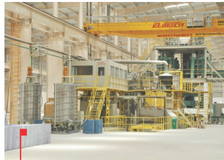
Ultra Modern Vacuum Vibro-Compression Compaction Technology
